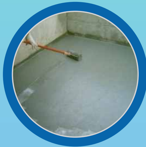
Cementitious Waterproof Coating Services
