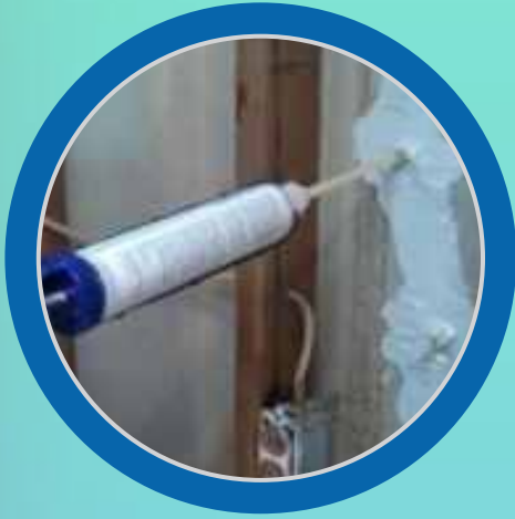
Polyurethane Injection Grouting Services
