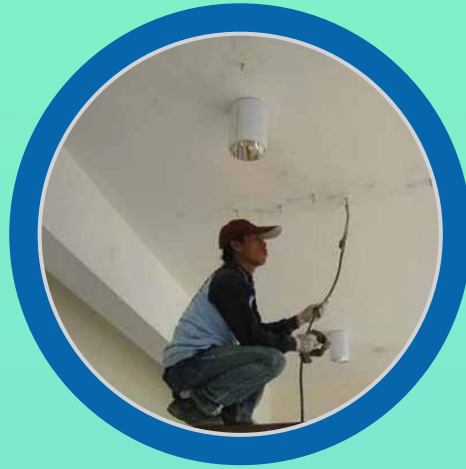
P.U Injection Grouting
